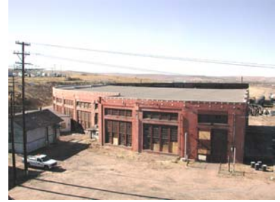
South back wall of the Roundhouse
