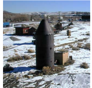
Building F and the incinerator
