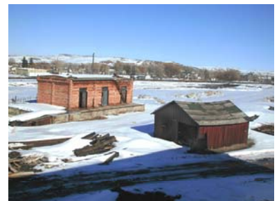
The Brick Store House (left) and Building E
